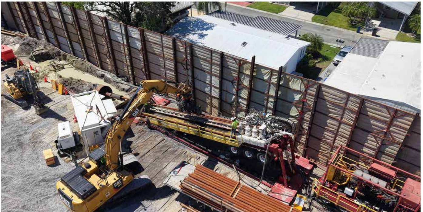
Aerial view of the Oldsmar work zone looking north. The horizontal directional drill is reaming through the casing.
