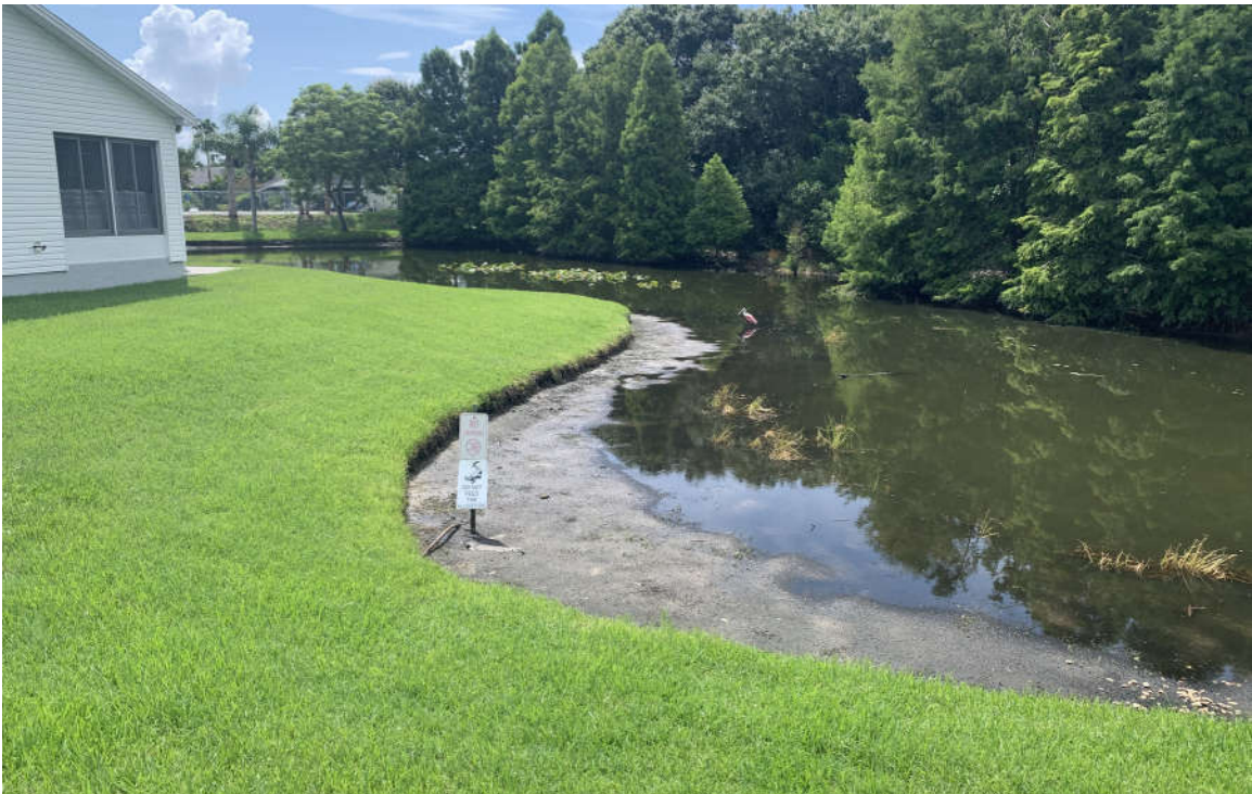
Erosion of bank (Basin 1)
