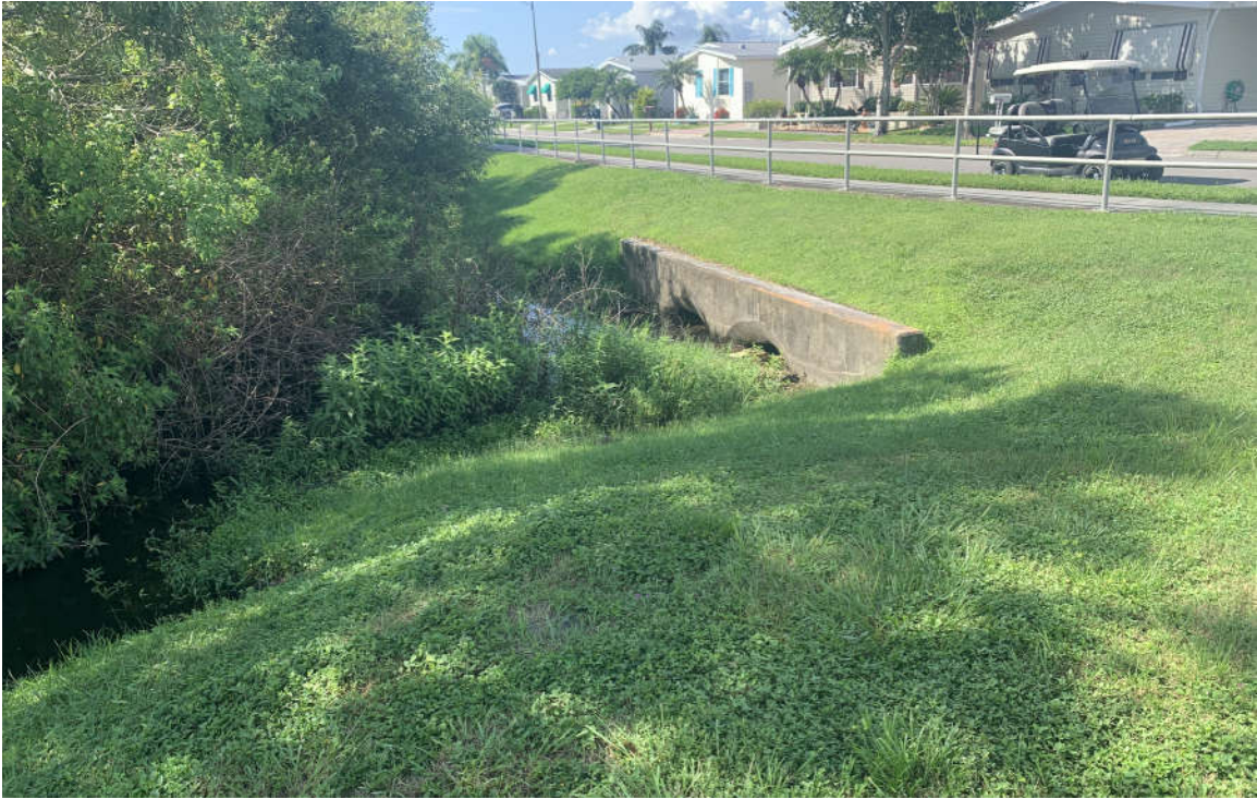
Continue to maintain vegetation (Northern spillway)
